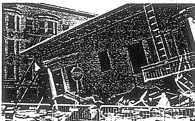
A collapsed building in the Marina District of San Francisco. Damage from the Loma Prieta earthquake.
